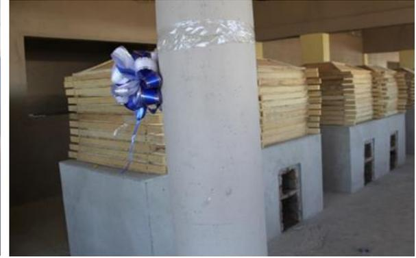
Figure 11: A picture of the fitted ovens in the smoking centre at Winneba
